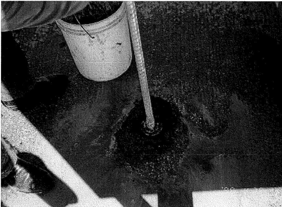
Figure 4.6 Patching the Hole After a Core being Extracted
